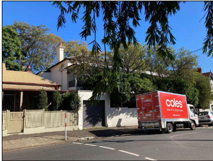
Figure 20: Nos. 16-18 Nicholson Street to the north of the site, a two-storey Victorian period building, now used as residential flats.
