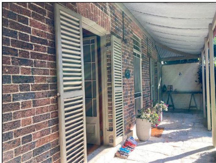
Figure 12: Front elevation showing verandah.
