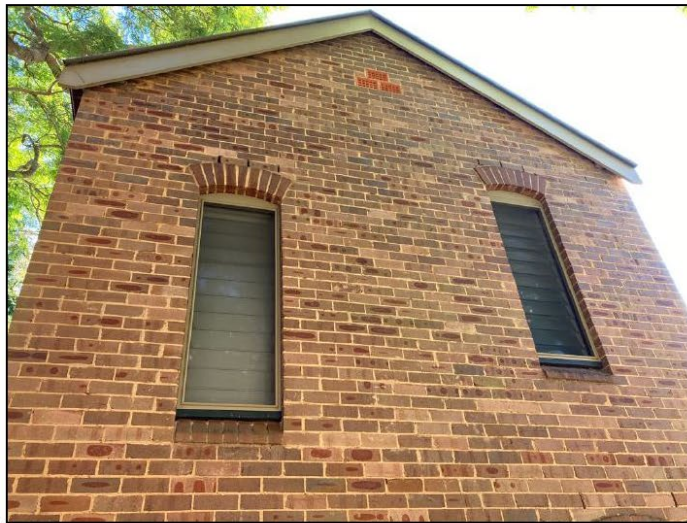
Figure 15: Southern elevation to the rear addition showing louvre window openings.
