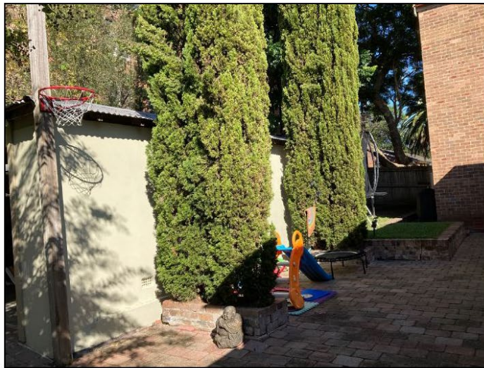
Figure 8: Looking towards the garage, partly concealed by vegetation.
