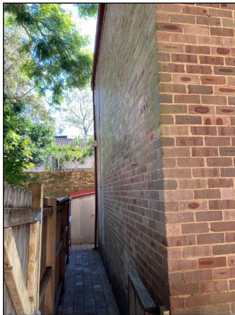
Figure 16: Western elevation to the rear addition.
