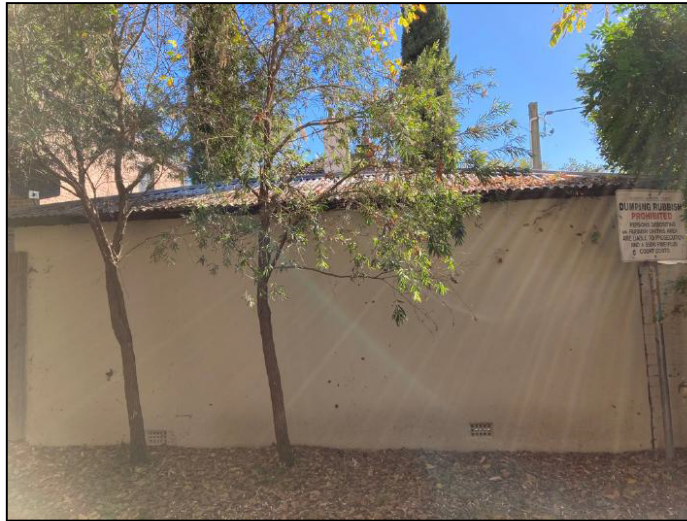
Figure 10: The existing garage as viewed from the entry to Origlass Park.
