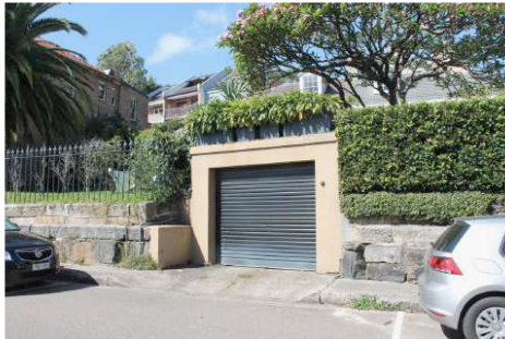
Figure 7.1 Garage to 36 Wharf Road
