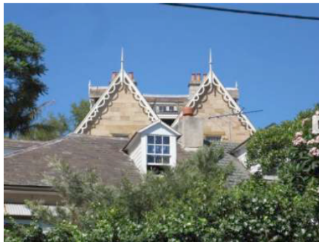
Figure 7.4 View to Clifton Villa over the subject site
