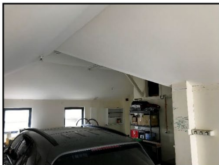
Figure 24. Interior of garage.
