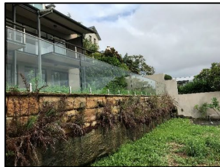
Figure 17. Sandstone wall to rear of subject site as viewed facing west.
