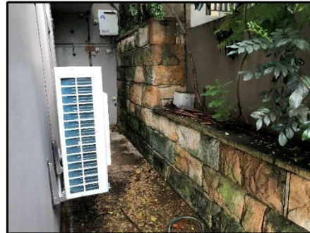
Figure 19. Western building line and boundary wall.
