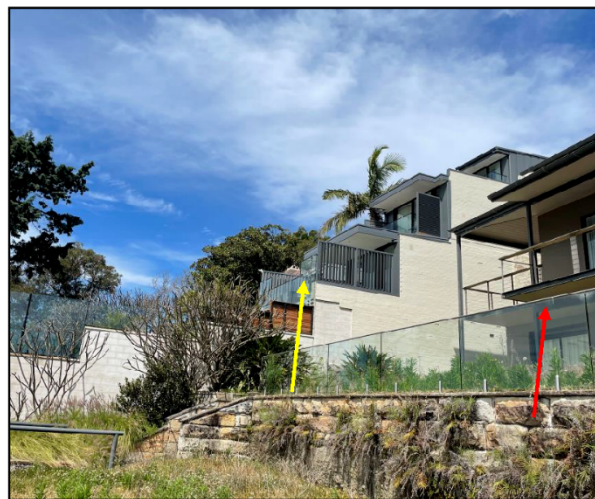
Figure 37. View towards 15a Wharf Road, Birchgrove (as indicated by the yellow arrow), depicting glazed balustrades, located adjacent to the subject site (as indicated by the red arrow). (Source: ESNH Design Pty Ltd).
