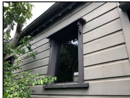
Figure 23. Timber window on eastern elevation of garage.
