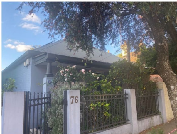
A grey metal roof opposite the Petersham Bowling Club.
