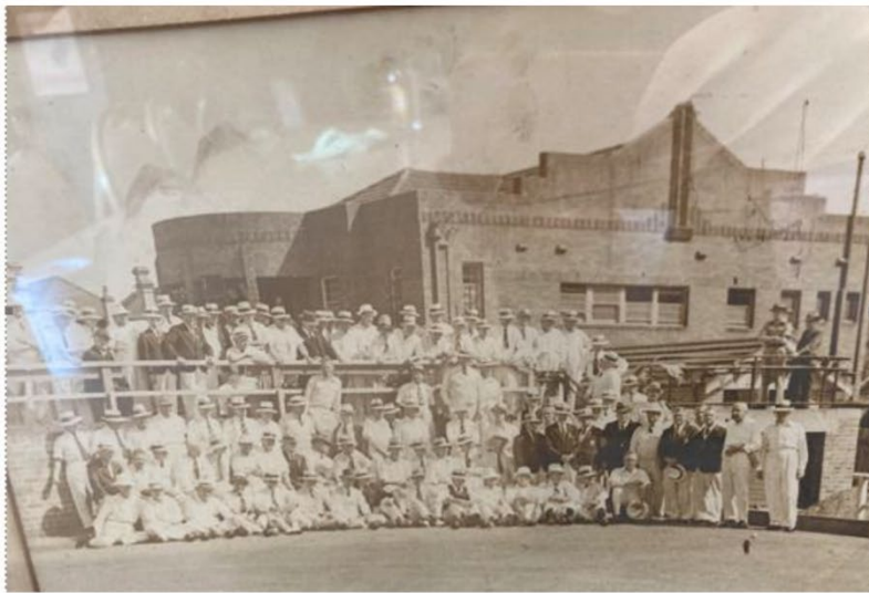
Shows façade facing Brighton Street, note gable end parapet
