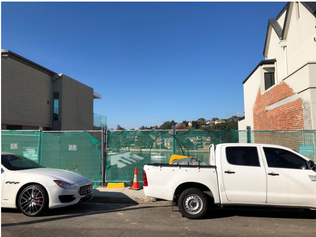
Figure 2: The subject site viewed from Louisa Road.
