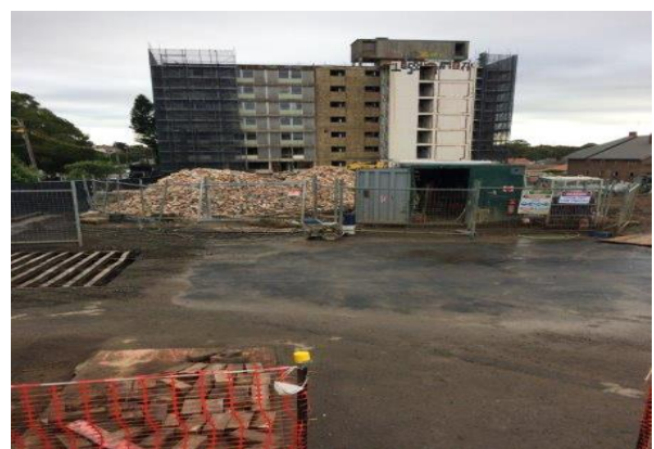
Demolition works on site
