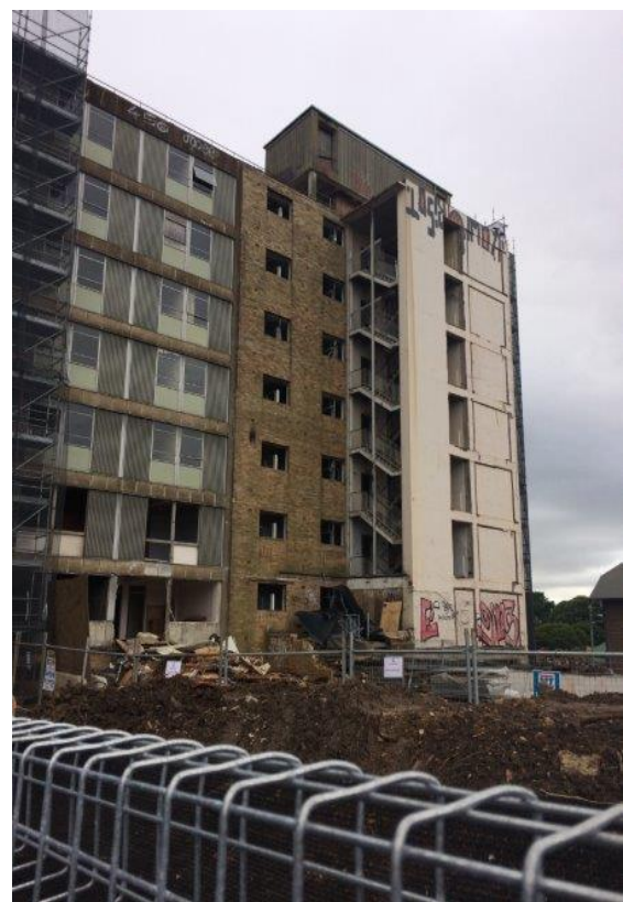
The former nurses' quarters will be demolished.
