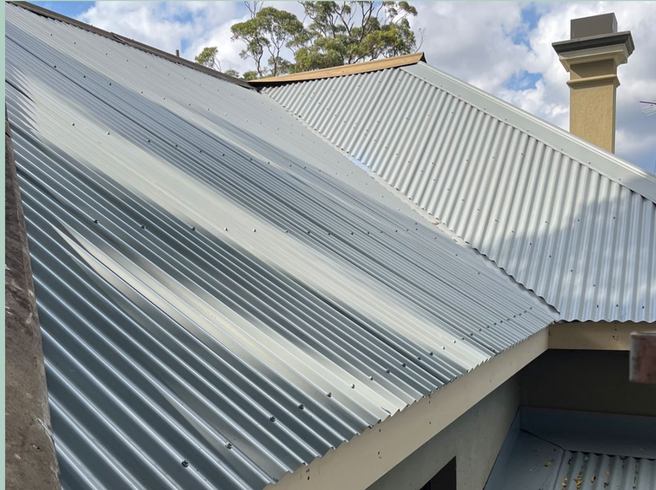
New roof sheeting
