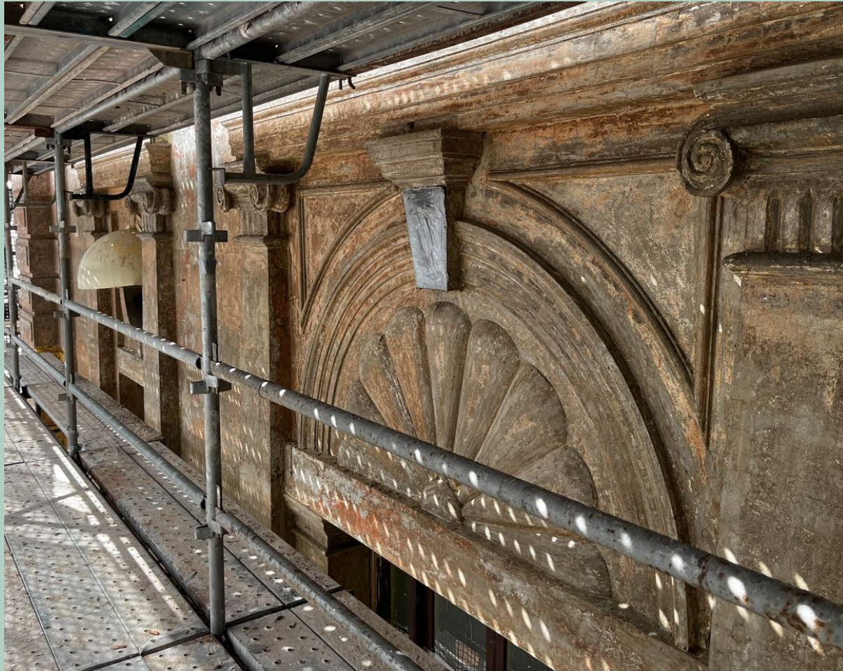
External paint stripping
