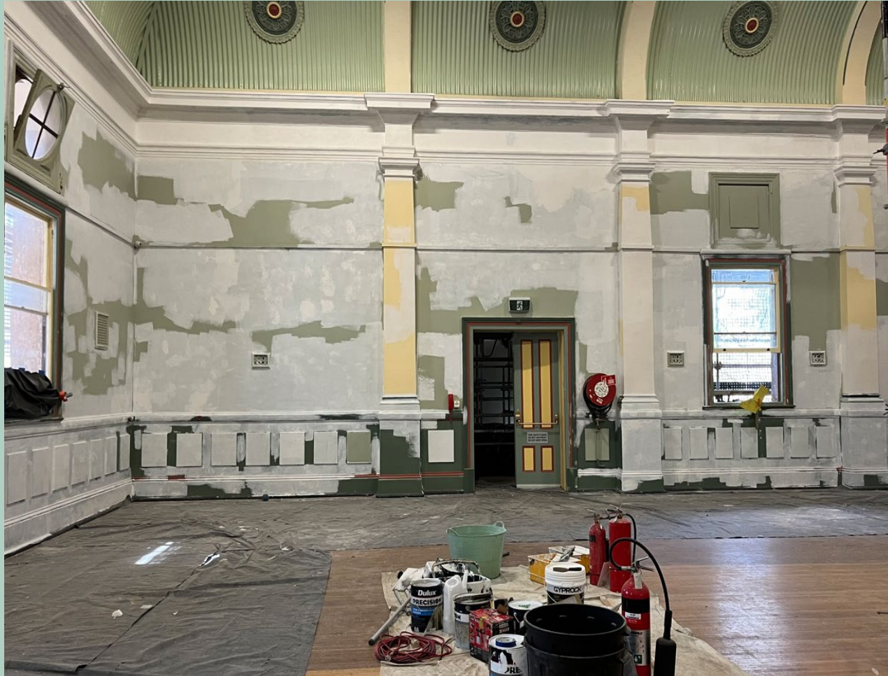
First Floor - Internal painting and patching in Town Hall
