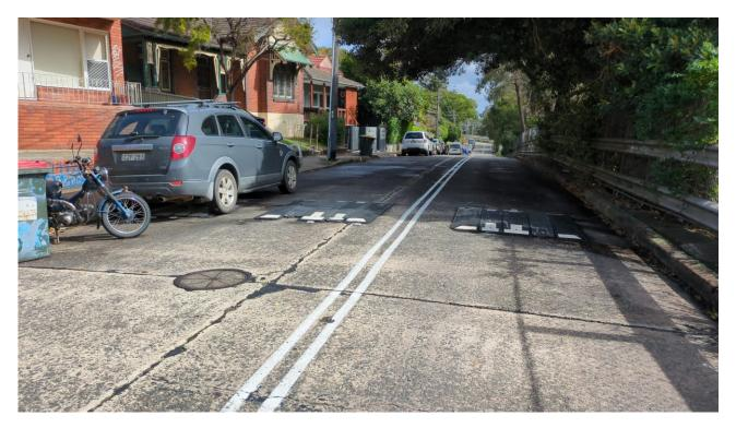
Replace signs due to damage & graffiti or missing (2 posts to be installed) Speed cushions to be installed to the same dimensions as the existing rubber cushions
