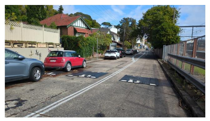
Replace signs due to damage & graffiti or missing (1 post to be installed) Speed cushions to be installed to the same dimensions as the existing rubber cushions
