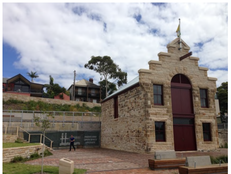
1880's Fenwick Stone Building at 2-8 Weston Street, Balmain
